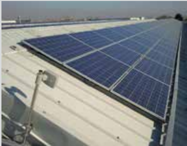
The orientable bracket gives the possibility to have the wiring completely hidden inside making all the installation procedures easy and fast too.
